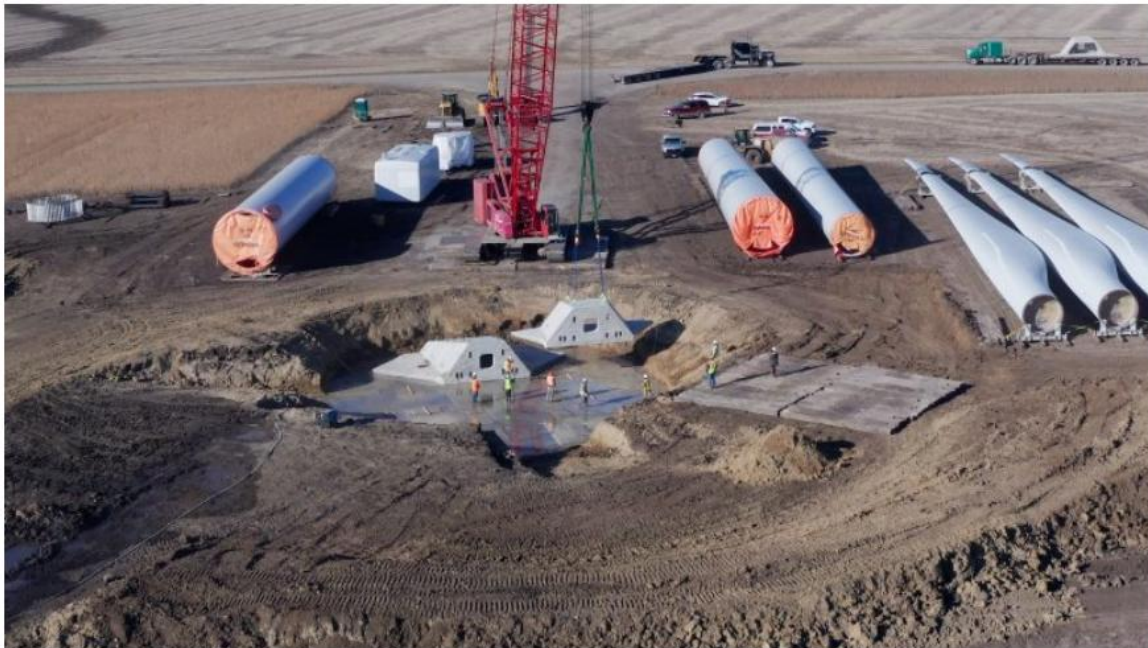
Plate A Turbine base construction pads (9 no. proposed). Note the scale of each of the three rotors relative to the construction workers.
